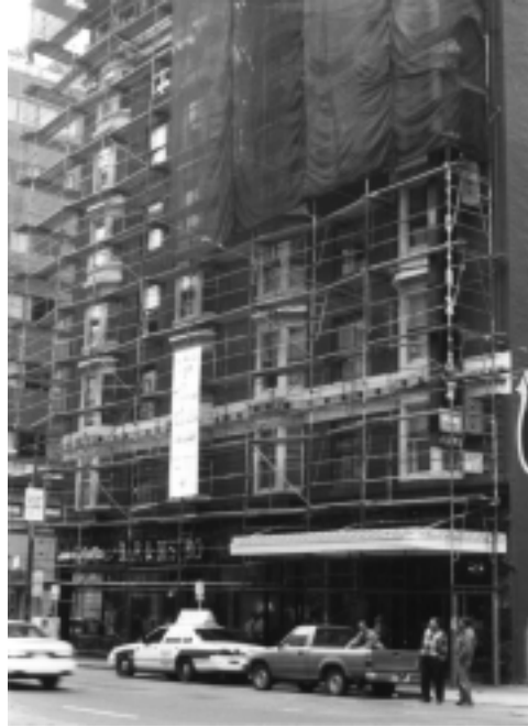
Figure 8-3. Renovation and expansion activities can expose occupants to products or particulates of construction.
