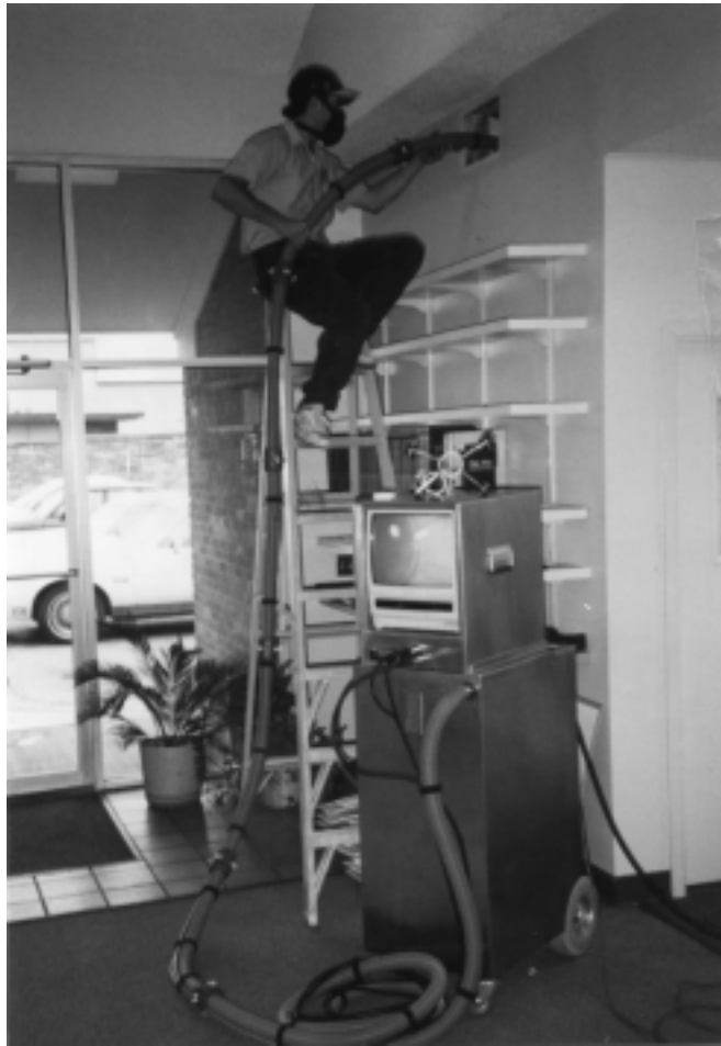
Figure 7-8. A video inspection of the ductwork. Courtesy: Clean-Aire Technologies.
